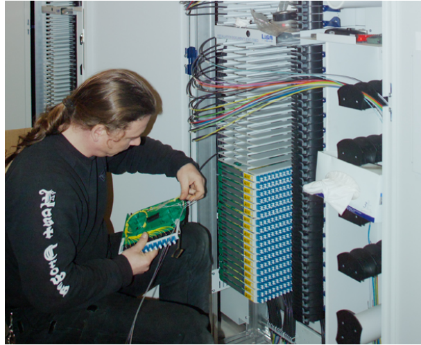
Figure 102: Splicing work on an ODF
