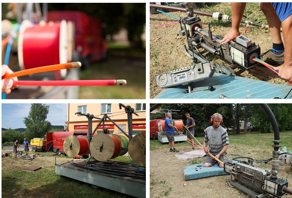
Figure 95: Air blowing of micro-ducts
