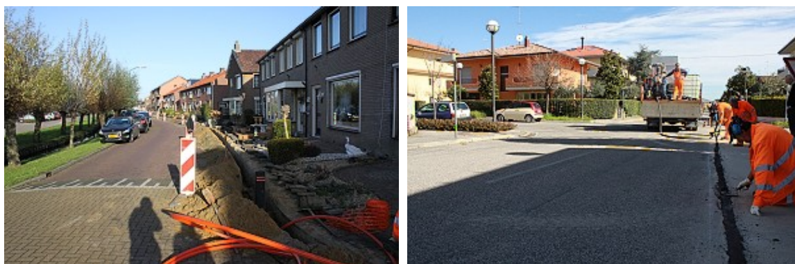
Figure 69: Conventional trenching vs microtrenching
