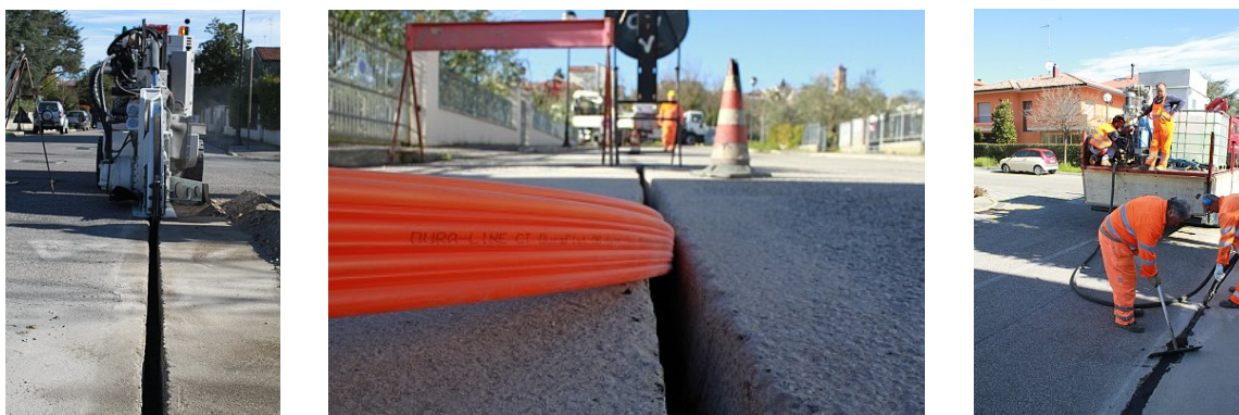
Figure 96: Micro-trenching deployment technique
