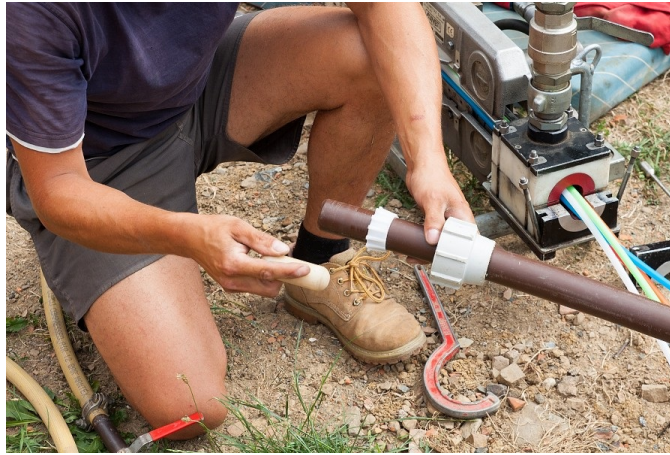
Figure 135: Preparation for shuttle blowing.
