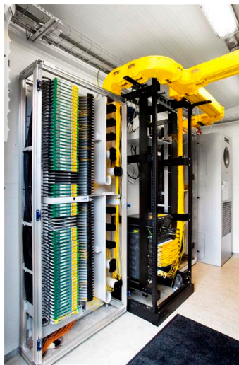
Figure 103: Active and Passive ODF's in a POP
