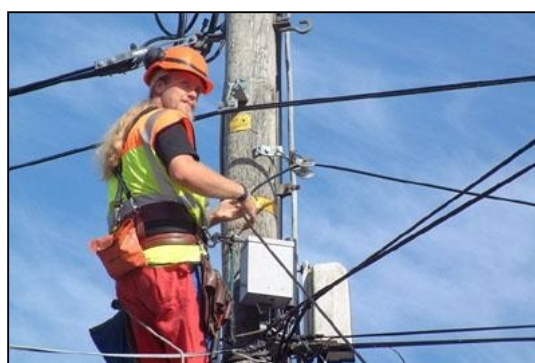
Figure 91: Aerial cable installation
