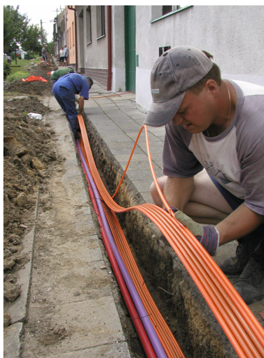
Figure 68: Deploying micro-duct infrastructure
