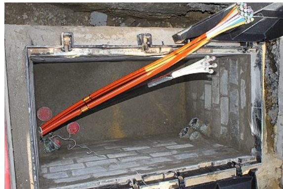
Figure 94: Bundles pulled in main duct
